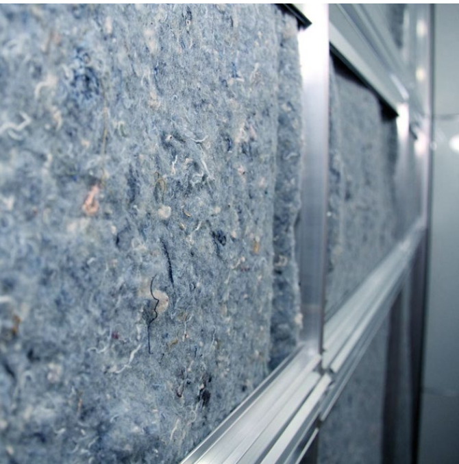
Denim insulation inside DIRTT solid wall frames.
