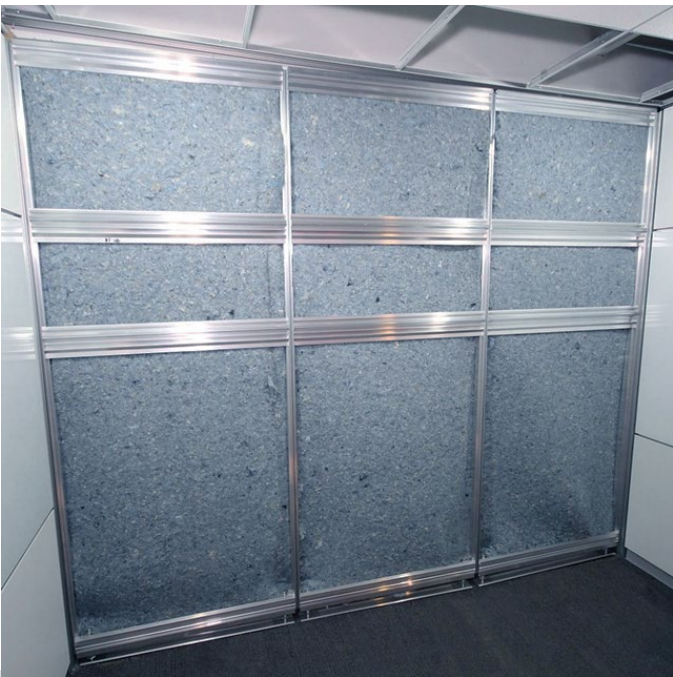
Denim insulation inside DIRTT solid wall frames.
